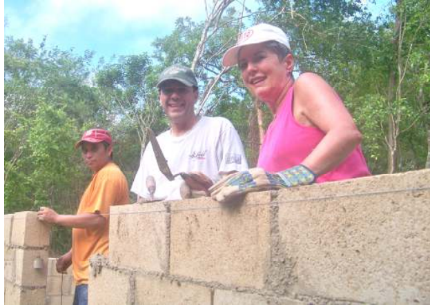
Laying block in Mexil
