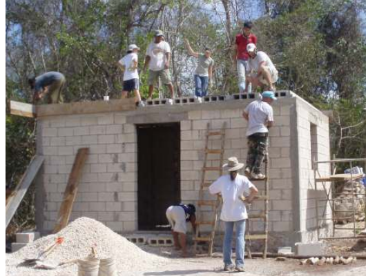
Northminster team members building a home in Huechenbalam
