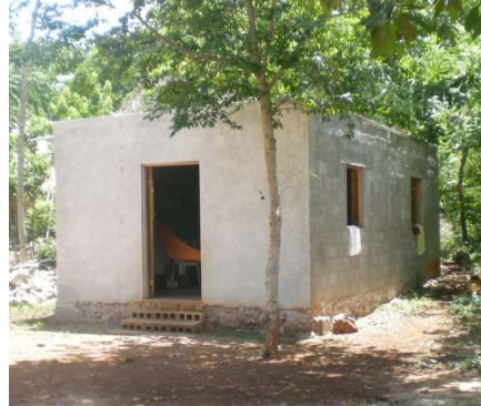
One of the new houses Acción helped build in Huechenbalam
