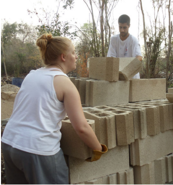
Fredericksburg team members move blocks to build a roof.
