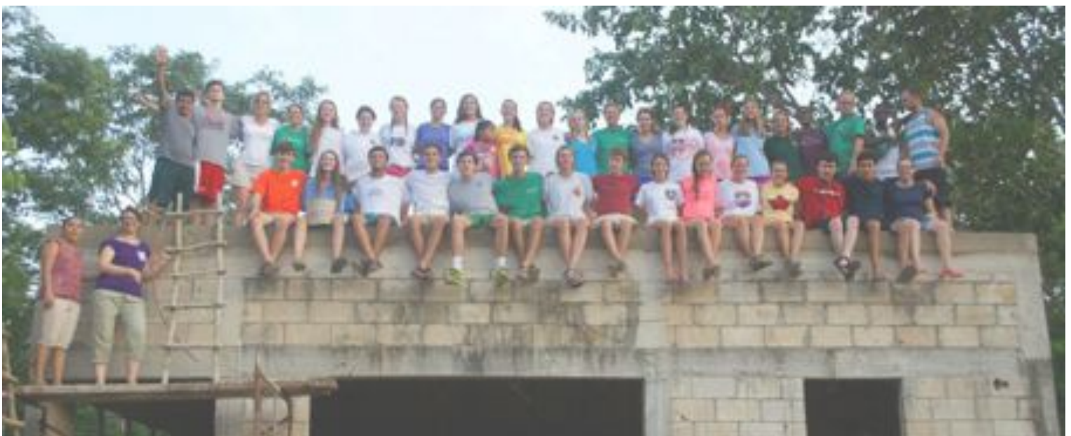
The team from First Presbyterian Church (Charlotte, NC) sitting atop the new kitchen facility at VIM that they helped construct .
